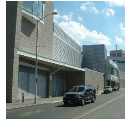
Service entrance on Commercial Street
