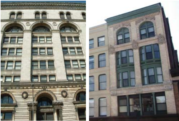
Façade articulation: Main Street
