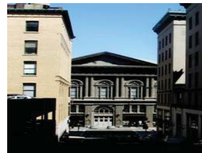
Prominent element: Walnut Street toward Main Street
