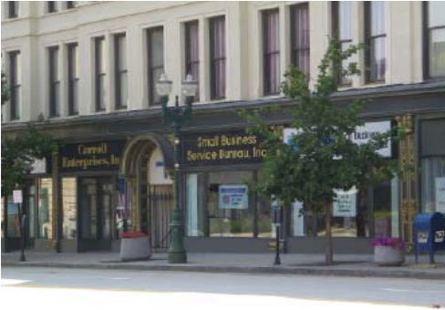
Street-level windows: Main Street
