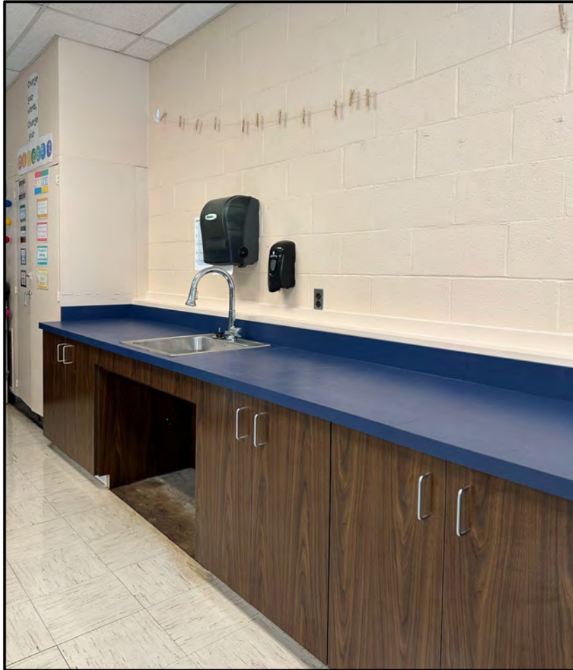
New casework & ADA sinks
