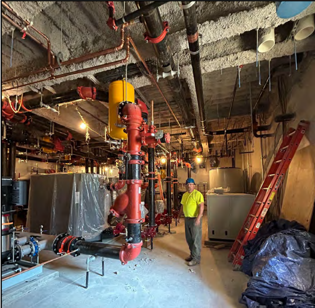
Boiler room - under construction
