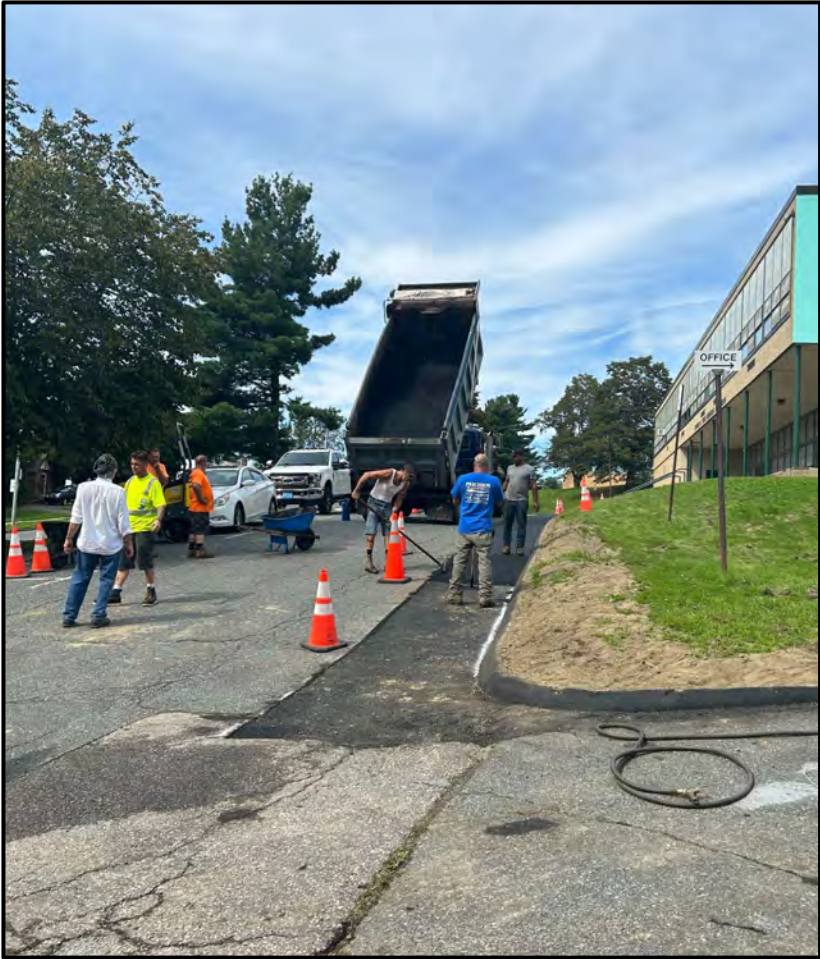
New curbs at drop-off
