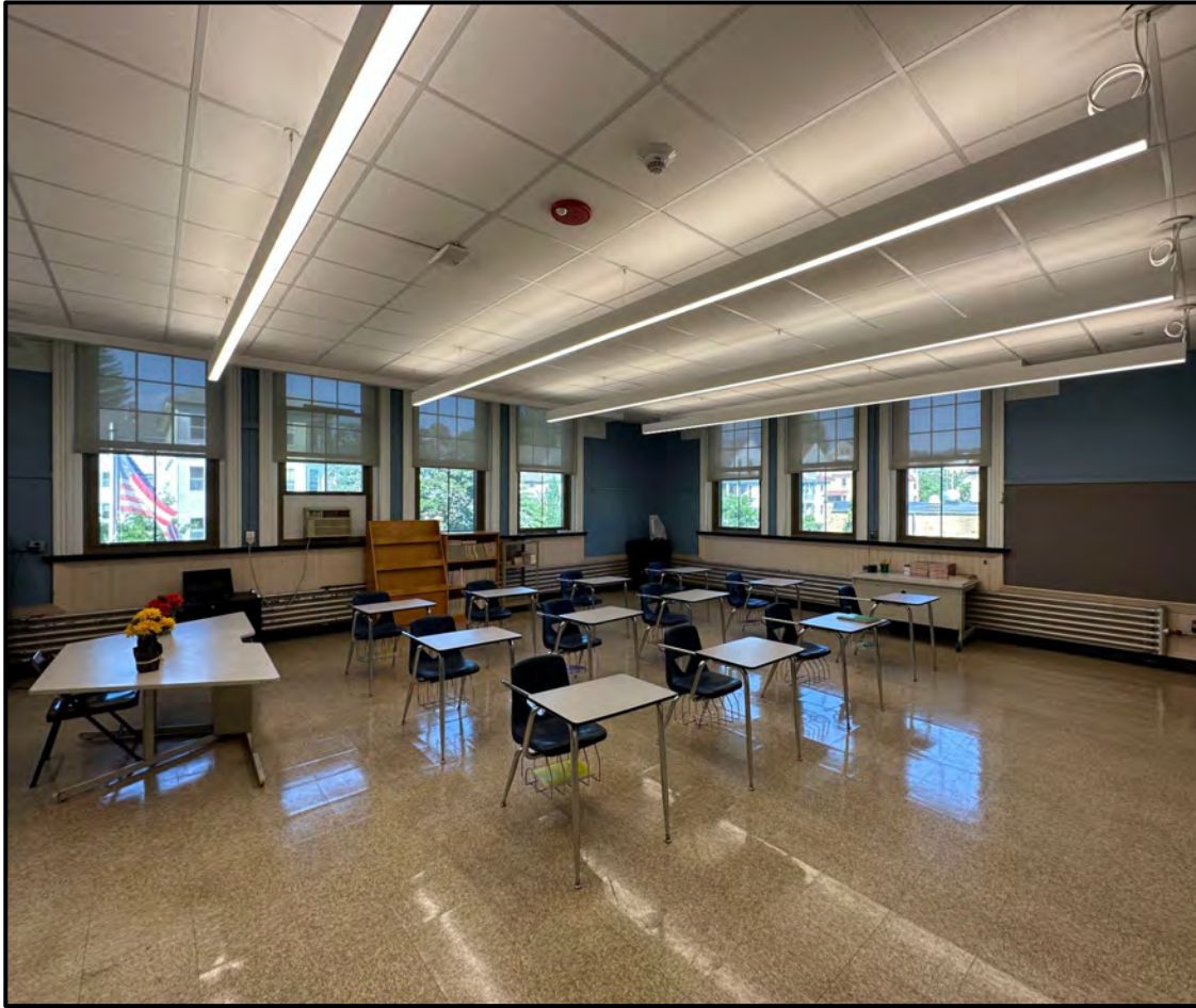
New ceilings, lighting, and sprinklers in all classrooms/interior spaces
