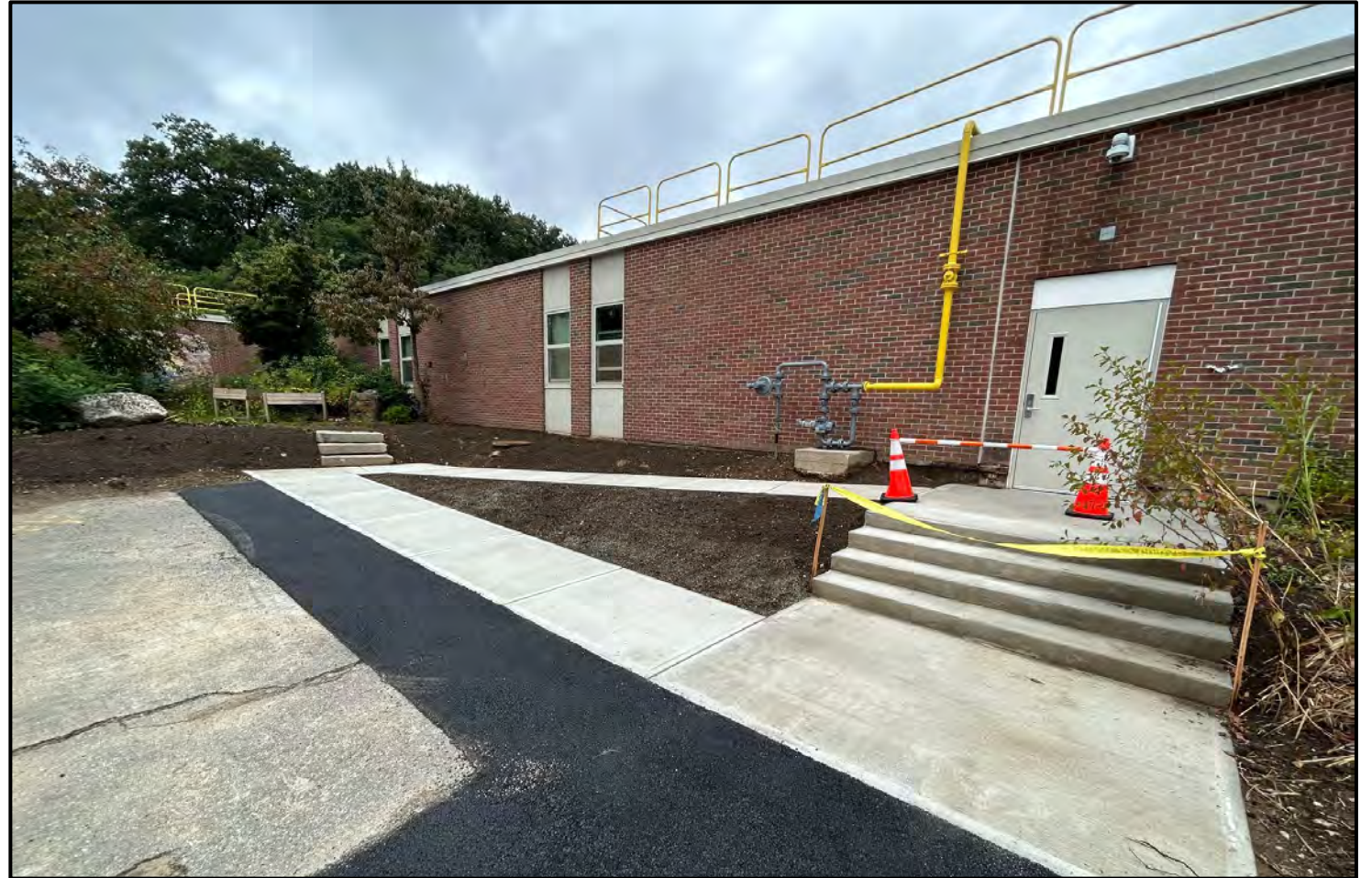
New exterior ramps & stairs
