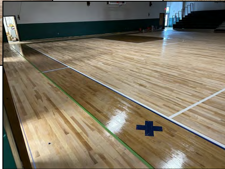
New bleachers, and entire space repainted
