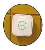
As part of the City project for the installation of a building energy management control system, the contractor is installing new sensors and digital thermostats. This is a significant upgrade from the older pneumatic thermostats. This will enable us to better respond to the client's needs as it relates to heating & cooling. This new system allows us to see what is happening and change what is needed in real time from a computer location.
