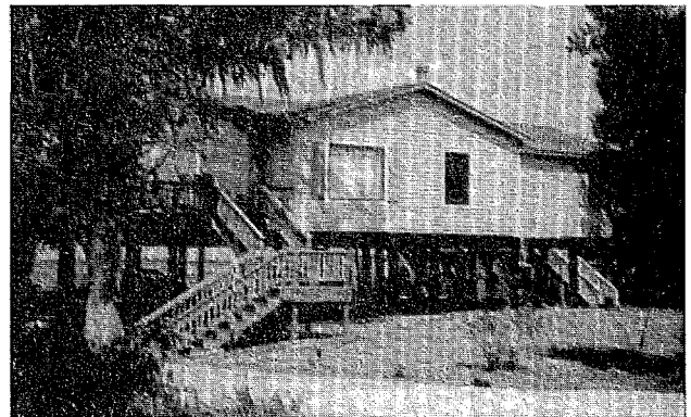
This 1,100-SF residential elevation project was accomplished in five days.
