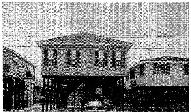
The home is set on the new pile foundation system.
