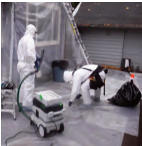
Lead paint abatement on a mid-20th century home.
