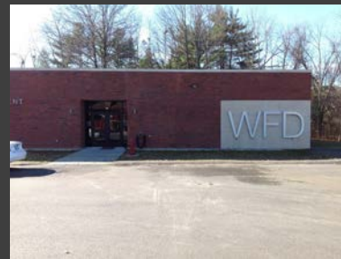
Fire Academy at HQ
