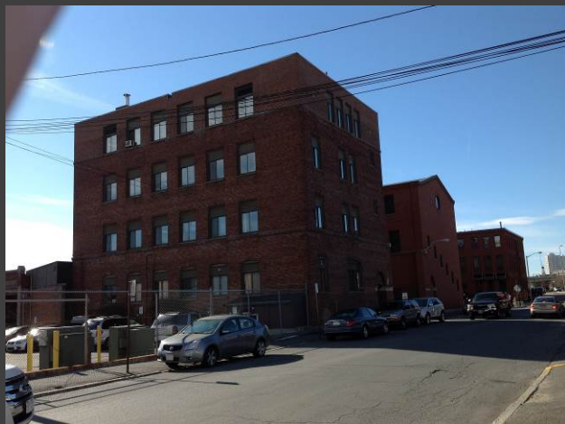
DPW Administrative Building – Water Operations
