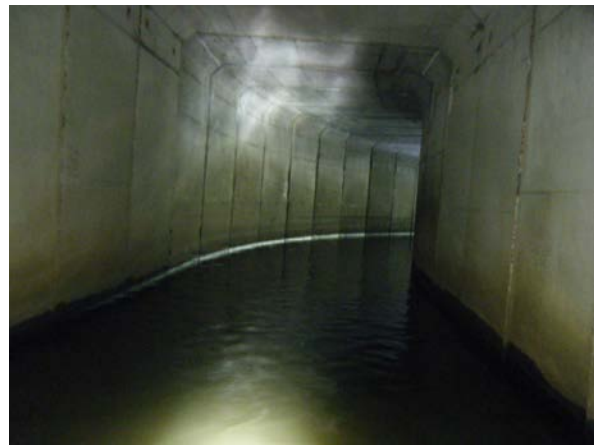
Mill Brook conduit extension under Worcester downtown.
