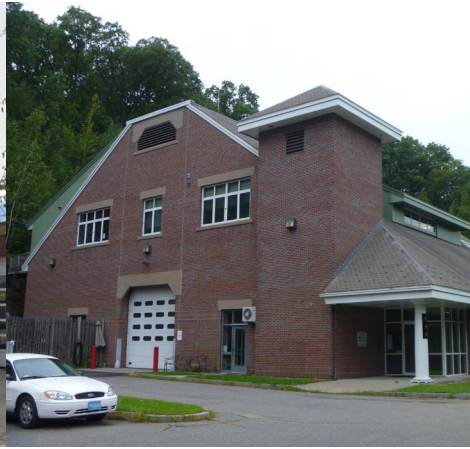
McKeon Road 80 Mckeon
