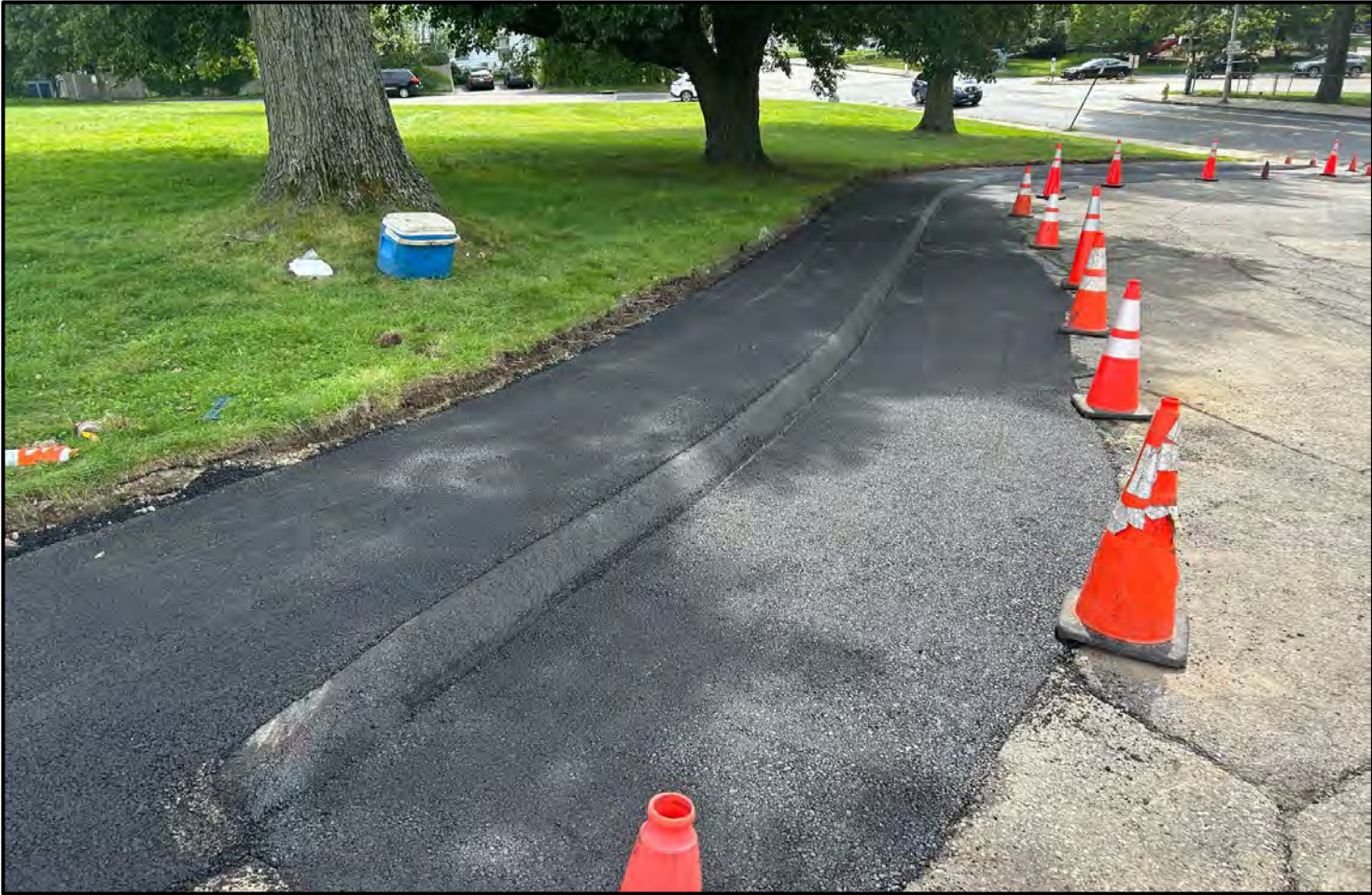
New sidewalk from Burncoat Street
