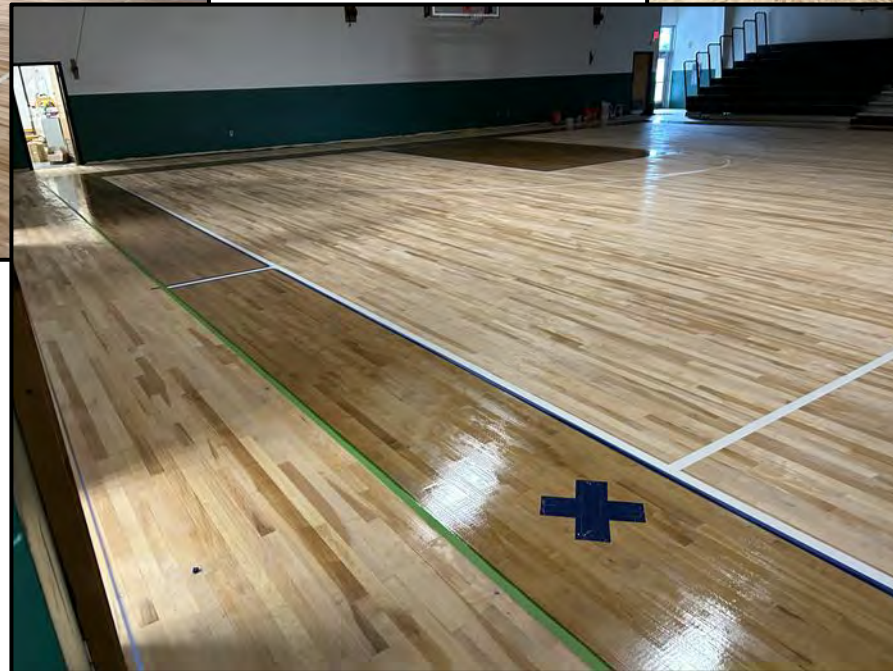
New bleachers, and entire space repainted
