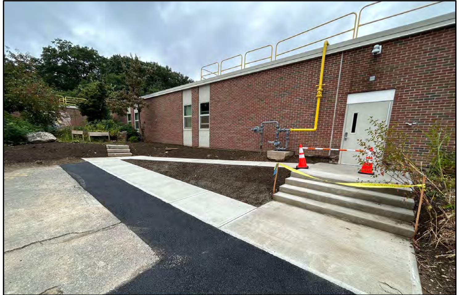
New exterior ramps & stairs
