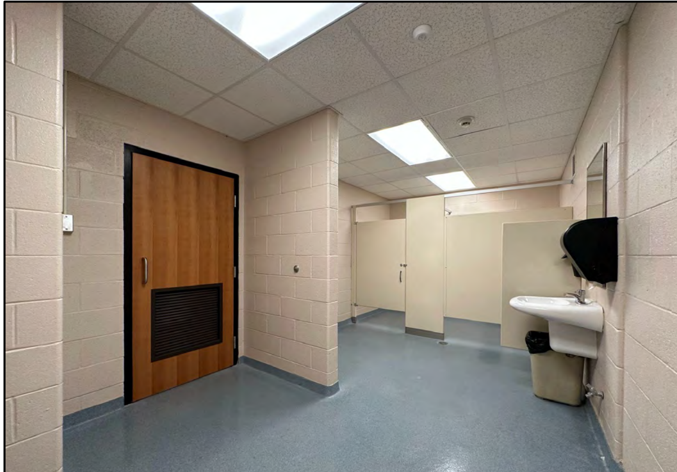
New bathrooms (typical)
