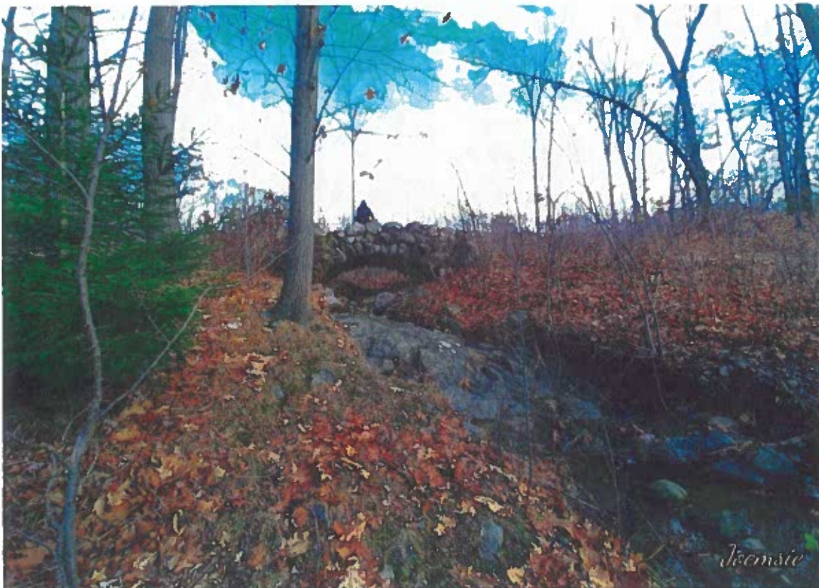
Arthurs Stone Bridge View Taken in 2020
