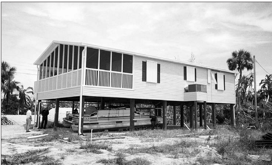
Figure 8-4. Manufactured home on a pile foundation.
