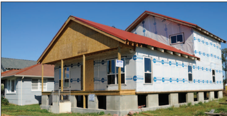
Figure 4-2. Redevelopment on a previously developed lot as part of the rebuilding process after Hurricane Katrina (Lakeview, LA)
