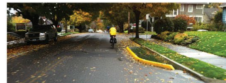
Curb Extension Bioswale Retrofit PORTLAND, OR
