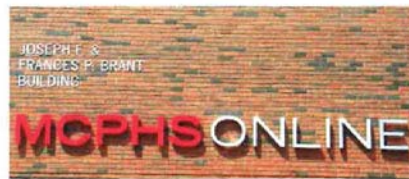
Building Identification Signage
