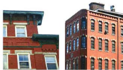
Distinctive roof line: Myrtle Street
