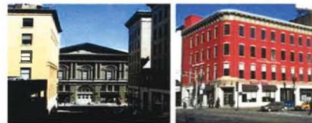
Prominent element: Walnut Street toward Main Street
