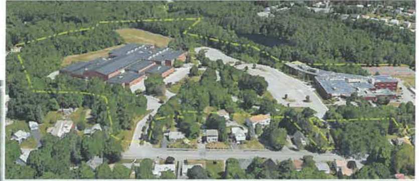
EXISTING AERIAL VIEW FROM SOUTH
