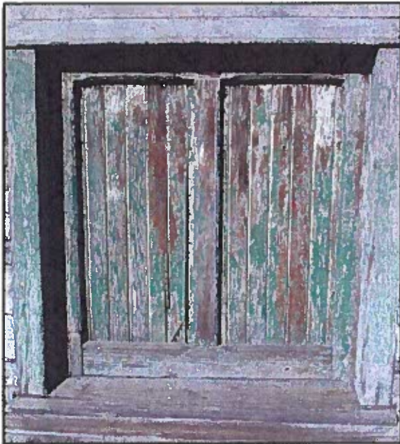
Photo 47: Original loft door of ell barn south facade. There are two original doors which should be retained and preserved. They are functional but have weathered surfaces and will need some carpentry repairs.
