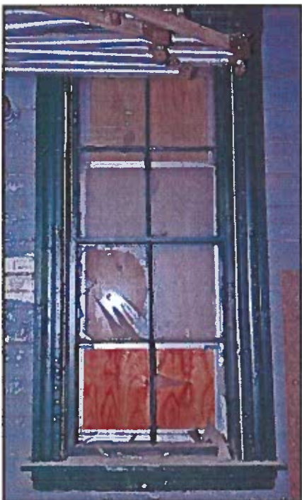
Photo 49: Interior side of first floor main barn window showing molded casings that should be retained and preserved. Sash are intact and can probably be retained with new glass and glazing.
