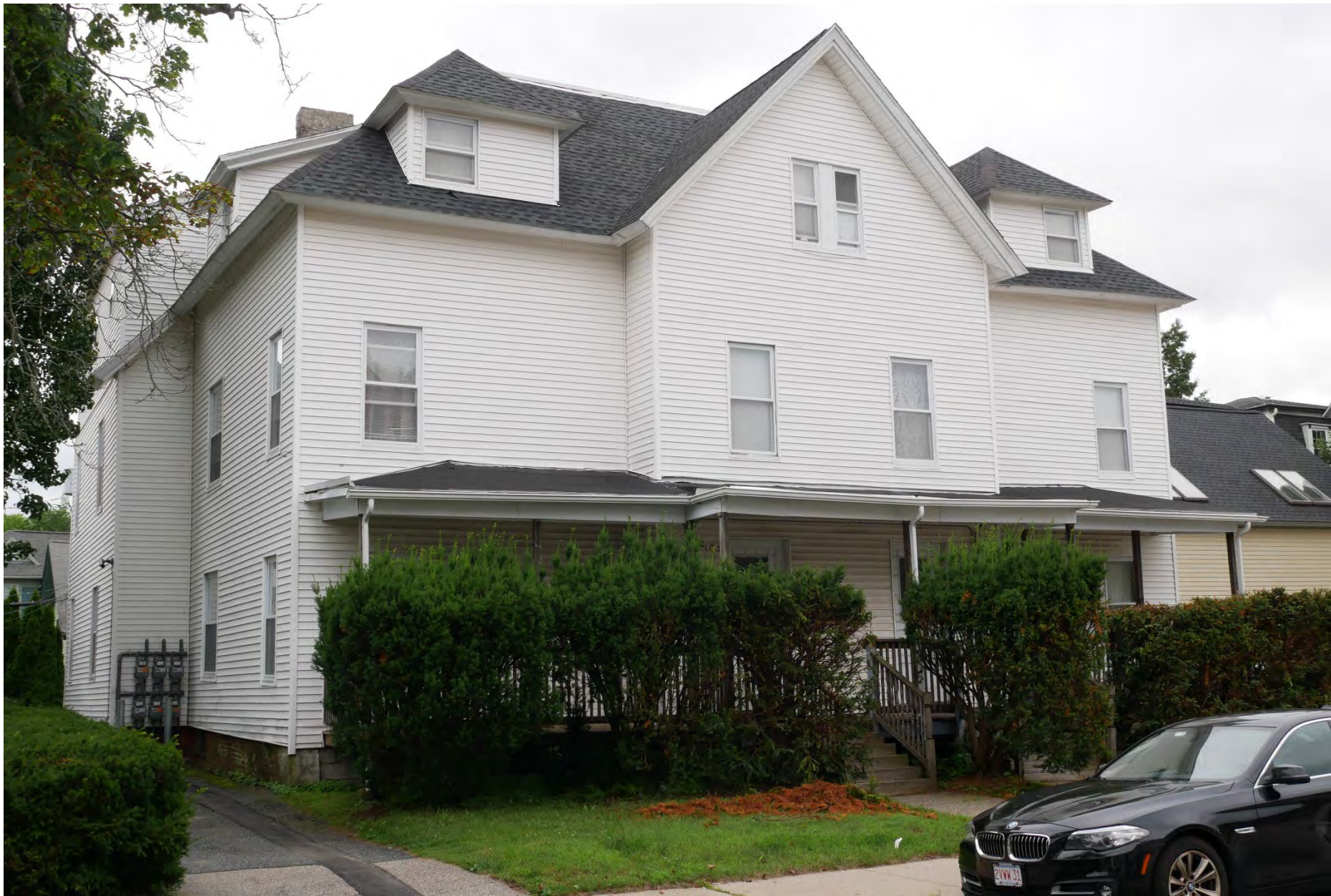
90. 101-103 Merrick Street, looking southeast. Integrity rating: poor
