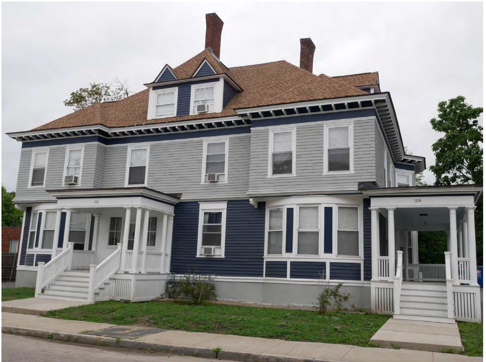
91. 102-104 Merrick Street, looking southwest. Integrity rating: good to very good
