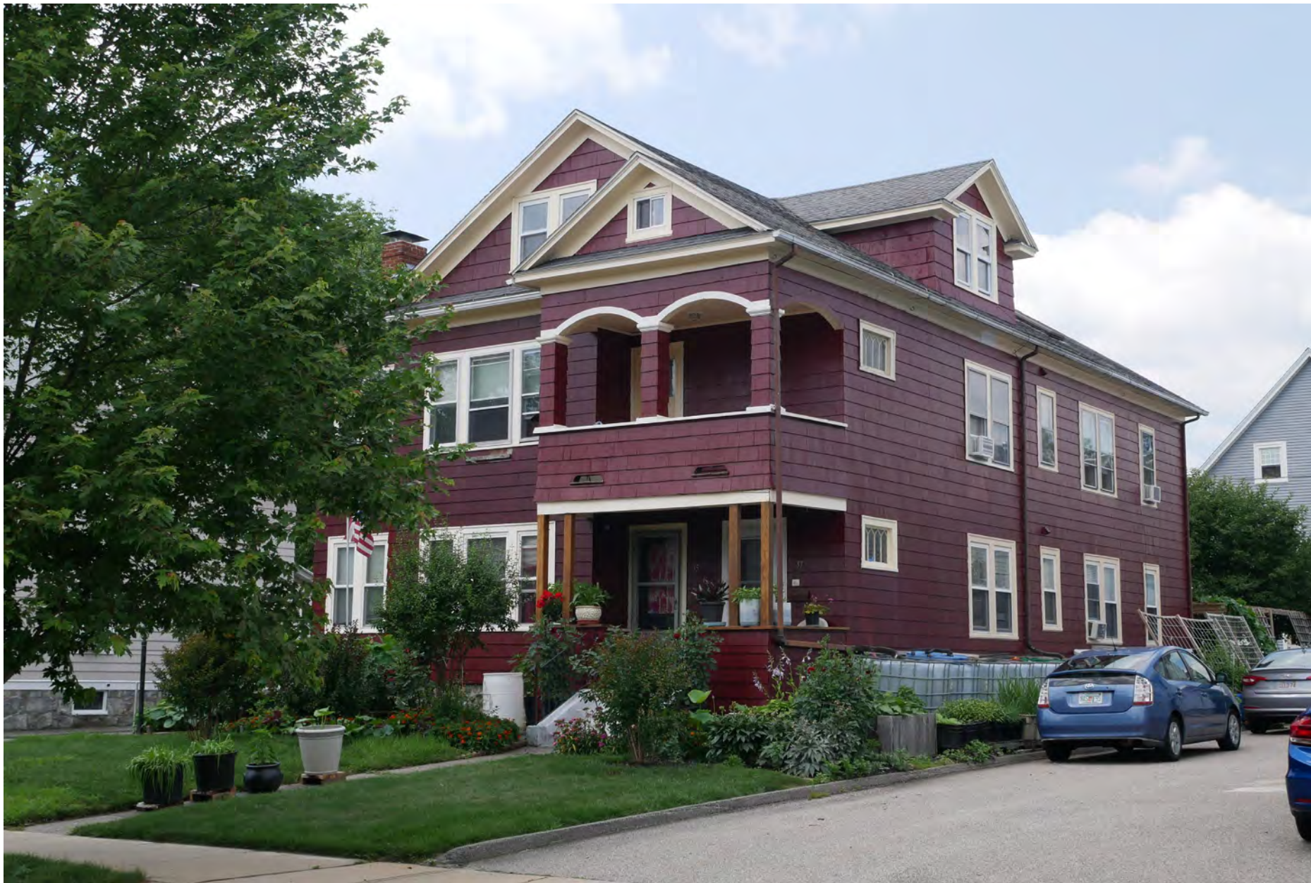
103. 35-37 Roxbury Street, looking southwest. Integrity rating: good
