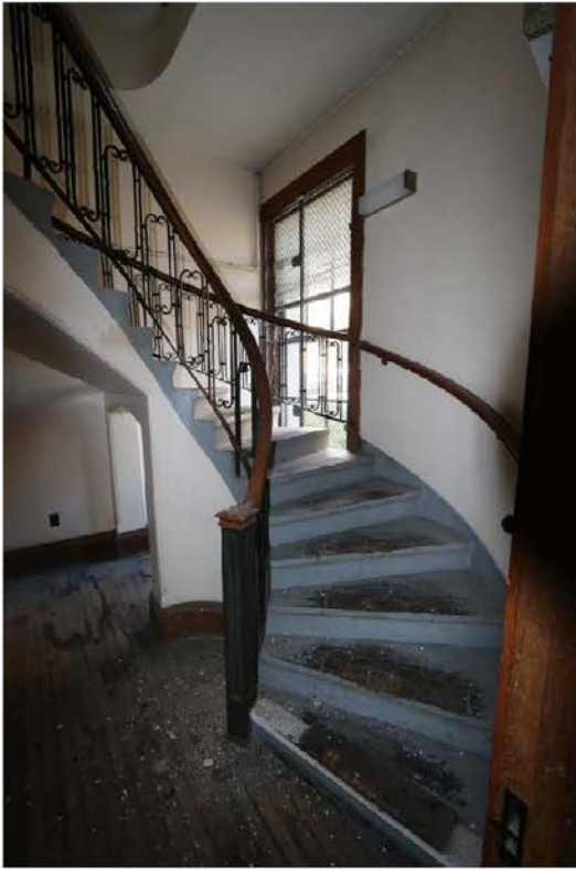
Figure 37: Spiral stairwell located in the northwest section of the building.
