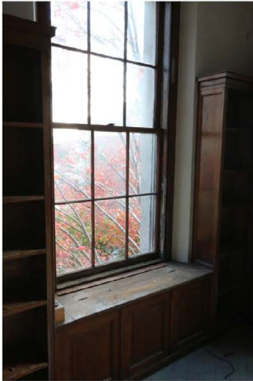
Figure 53: 1878 addition, view toward Main Street.
