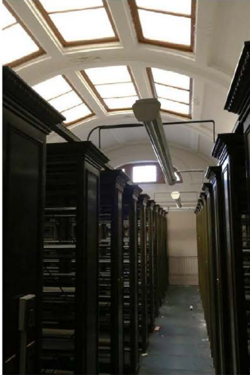
Figure 54: Library and skylights within the 1878 Addition.
