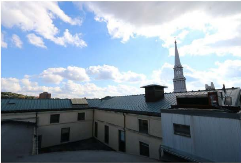
Figure 16: Interior Courtyard from Roof (View of neighboring First Unitarian Church)
