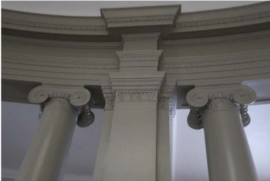
Figure 35: Molding detail, second floor lobby.
