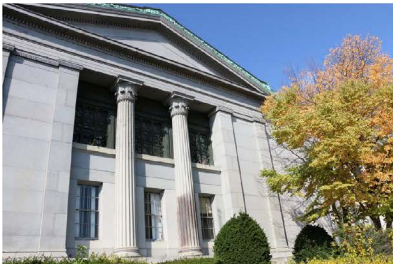
Figure 7: Updated 1898 Façade on the Original 1845 Building (Facing Main Street)
