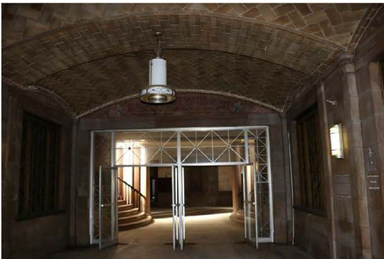
Figure 26: First floor entry, looking toward lobby
