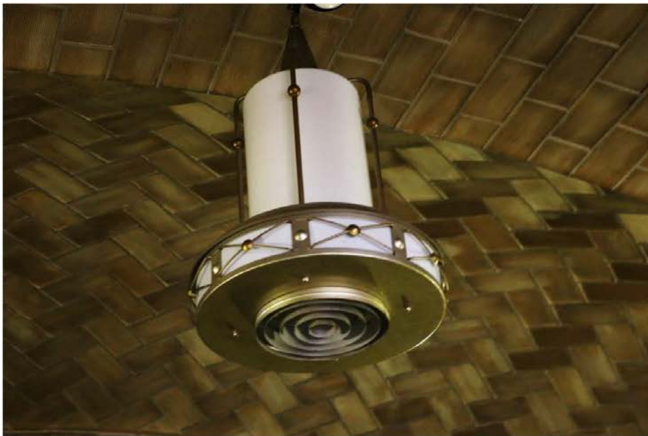
Figure 28: Light fixture and ceiling detail in first floor entry
