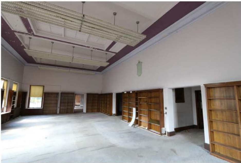
Figure 52: 1878 addition to the south side of the building.
