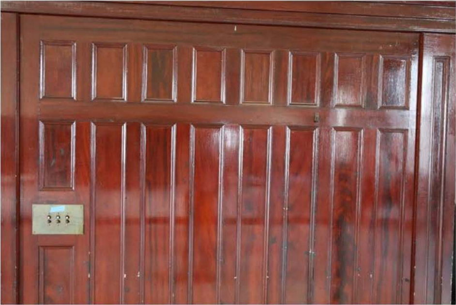
Figure 47: Southwest courtroom – wall paneling
