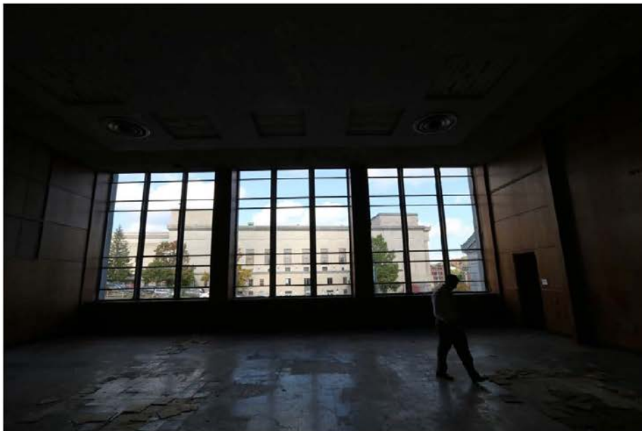
Figure 66: View of Worcester Auditorium from courtroom
