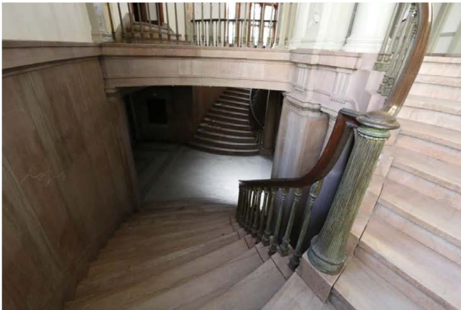
Figure 30: Main staircase, looking down toward first floor
