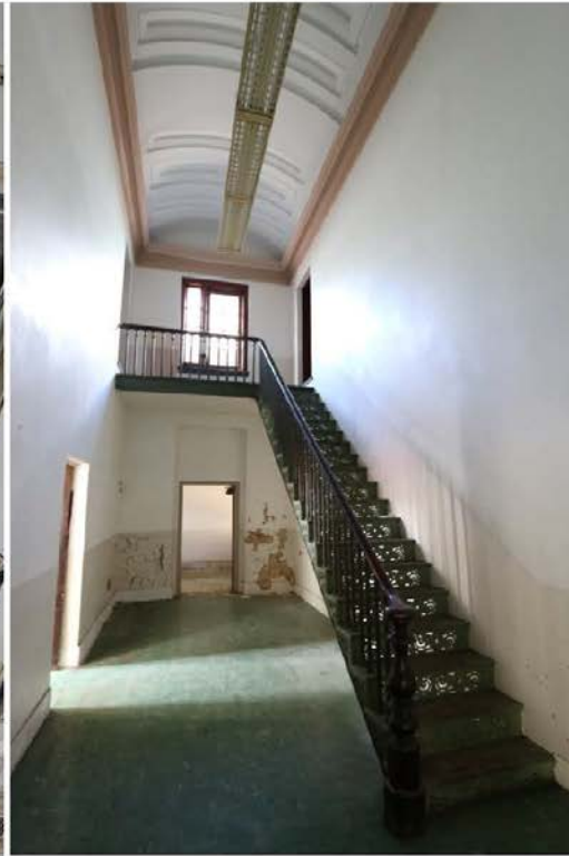
Figure 49: Stairwell outside of the southeast courtroom.
