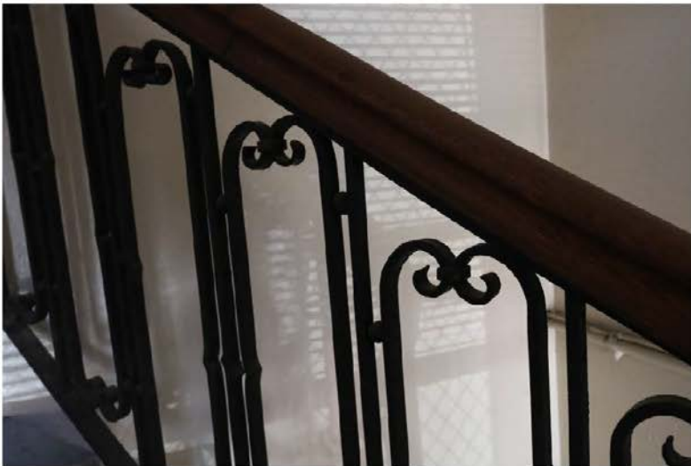
Figure 38: Detail, spiral stairwell
